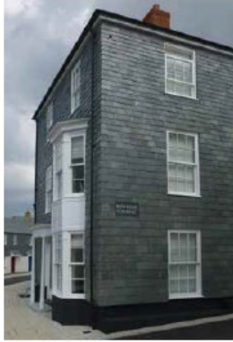
Hung slate building
