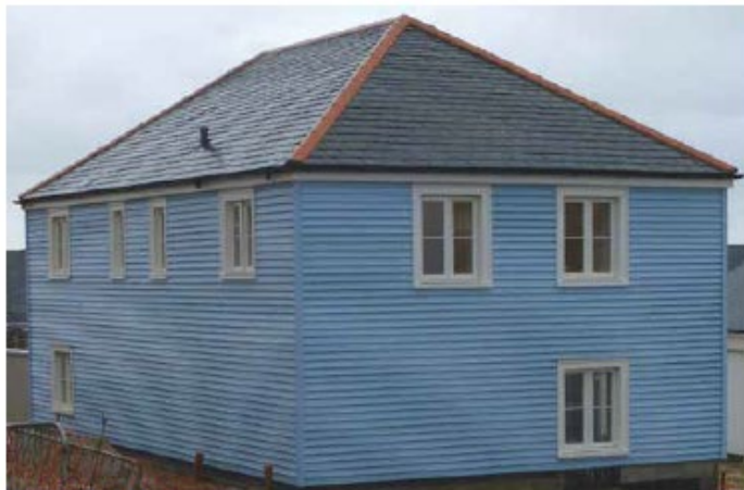
Painted timber building
